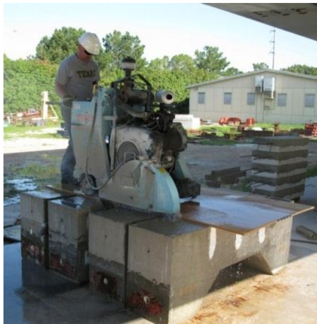
Figure 5.2: Sawcuts in Progress
