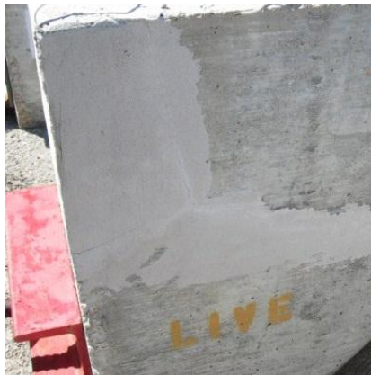
Figure 5.87: Specimen 3.4, Efflorescence at Live End Corbel and Pourback Cracks
