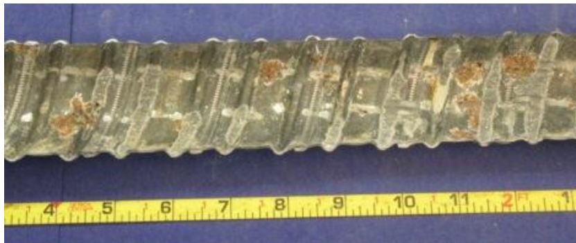
Figure 5.25: Specimen T.2, Corrosion Along Gouges on Bottom Half of North Duct
