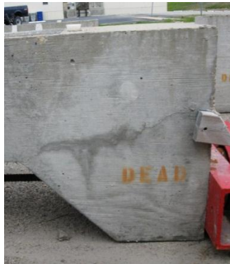
Figure 5.63: Specimen 3.1, Efflorescence at Dead End Corbel Crack
