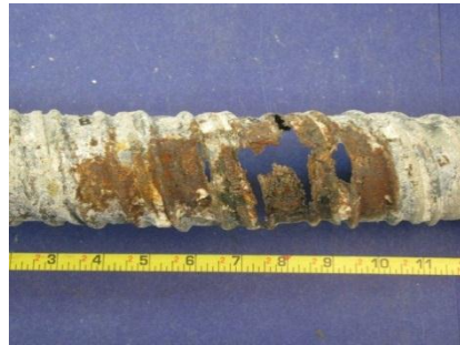
Top of South Duct
