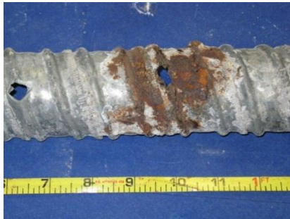
Top of North Duct
