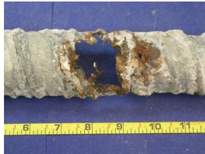
Top of South Duct
