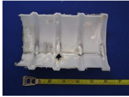
Top of South Duct
