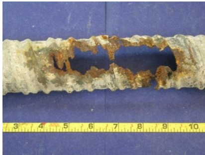
Top of North Duct
