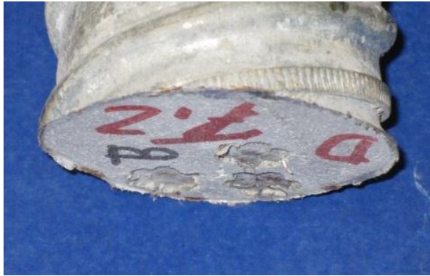
Figure 5.30: Specimen T.2, Debonded Strands in South Anchorage
