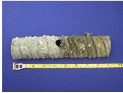
Top of South Duct
