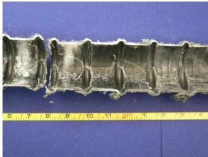
Top of North Duct
