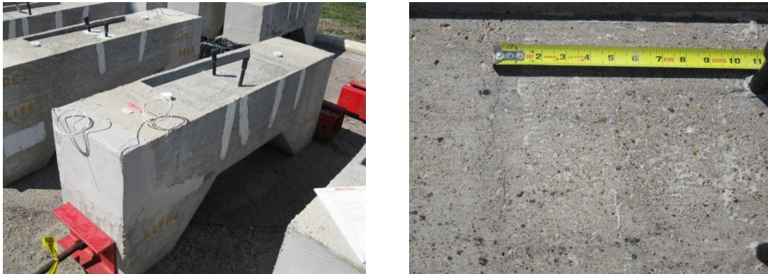
Figure 5.86: Specimen 3.4 Overall (Left) and Discoloration Around Surface Cracks (Right)
