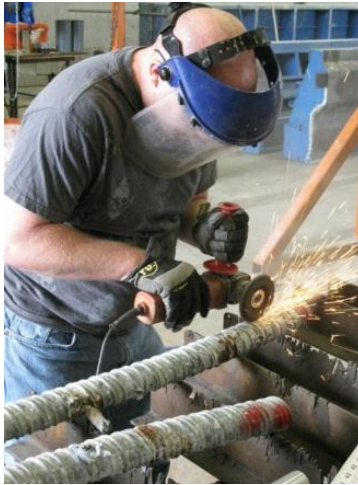
Figure 5.9: Removing Ducts Using Electric Grinder
