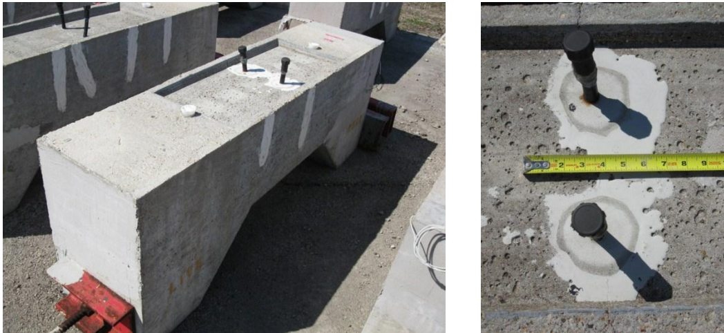
Figure 5.14: Specimen T.1 Overall (Right) and Grout Vents (Left)
