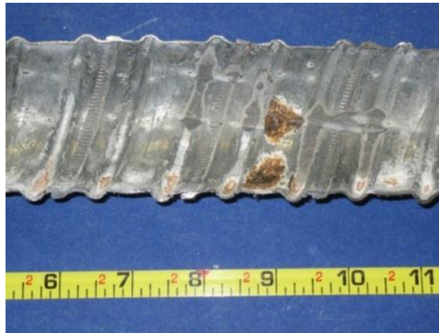
Figure 5.16: Specimen T.1, Corrosion Along Gouges on Bottom Half of North Duct
