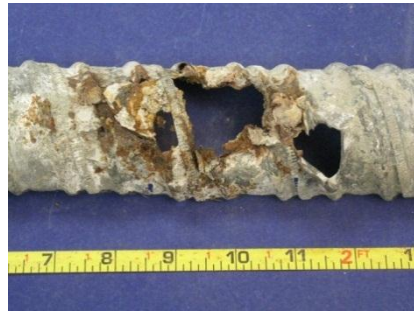
Top of South Duct
