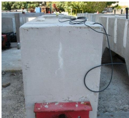
Figure 5.107: Specimen 7.1, Efflorescence Around Crack on Live End
