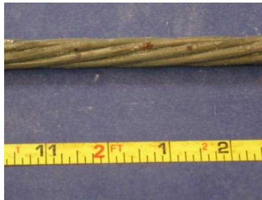
Figure 5.26: Specimen T.2, North Duct Strand Showing Pitting Near Midspan
