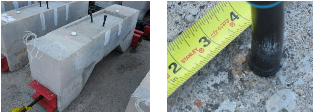
Figure 5.96: Specimen 4.2 Overall (Left) and Discoloration Around North Grout Vent (Right)
