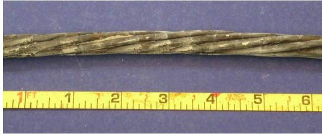
Figure 5.56: Specimen 2.4, Lines in Strand Discoloration
