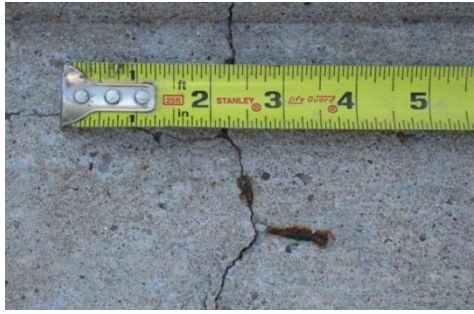
Figure 5.53: Specimen 2.4, Corroded Wire Tie at Top Surface
