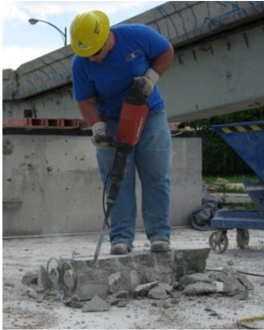
Figure 5.6: Main Autopsy Block Chipping in Progress
