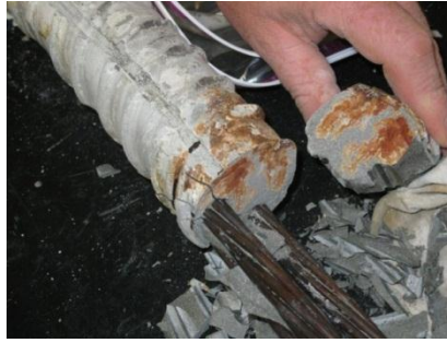
Figure 5.36: Specimen 1.2, Corrosion Staining Within South Grout
