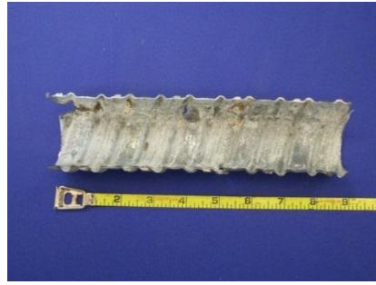
Top of South Duct
