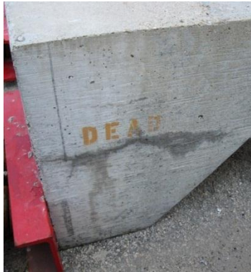
Figure 5.97: Specimen 4.2, Efflorescence and Moisture around Dead End Corbel Crack
