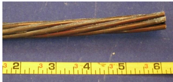
Figure 5.37: Specimen 1.2, Possible Dezincification Near Strand End
