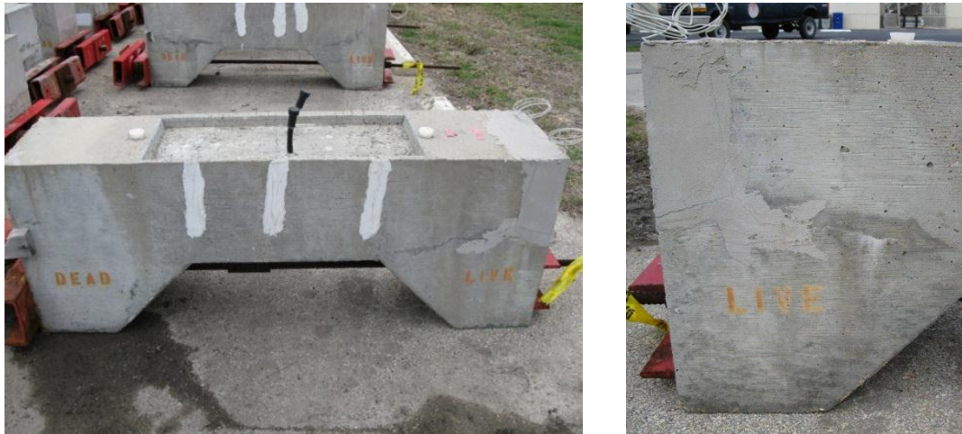
Figure 5.74: Specimen 3.2 Overall (Left) and Efflorescence at Live End Corbel Crack
