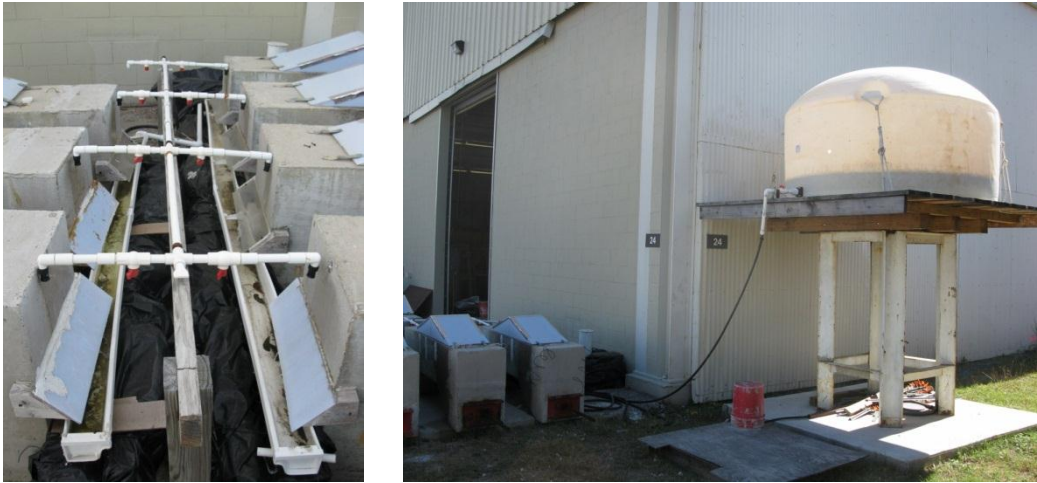
Figure 3.2: Repaired Drippers in Operation (Left) and New Tank System (Right)
