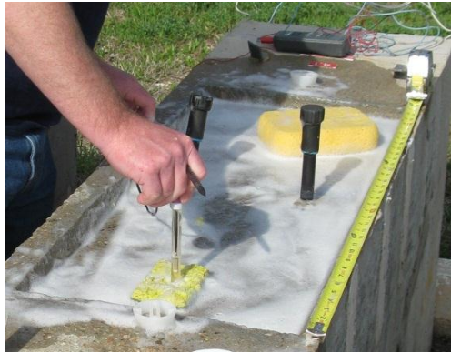
Figure 3.3: Half-Cell Potential Measurements in Progress
