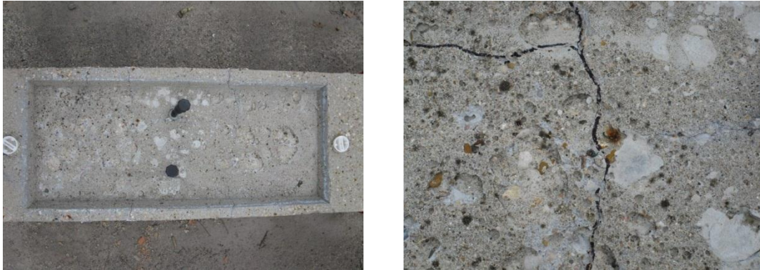
Figure 5.62: Specimen 3.1 Top Surface (Left) and Corroded Wire Tie at Top Surface (Right)
