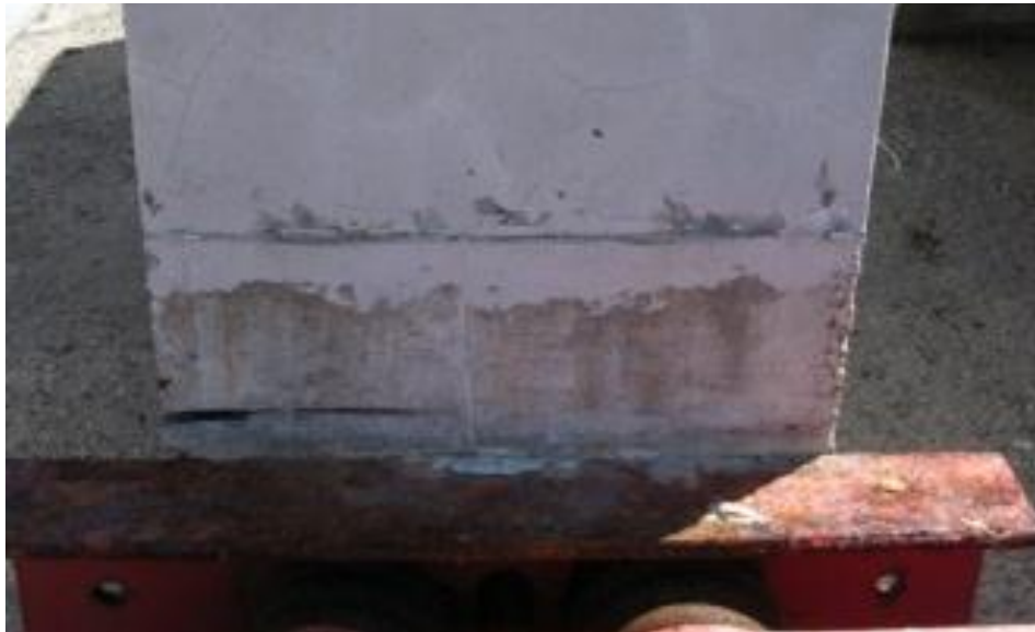
Figure 5.23: Specimen T.2, Separation and Delamination Around Dead End Pourback
