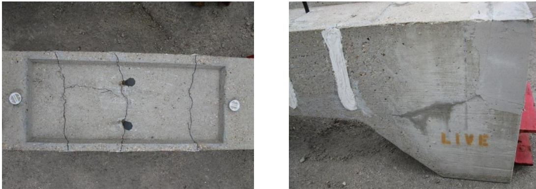
Figure 5.33: Specimen 1.2 Top Surface (Left) and Leakage at Live End Corbel Crack (Right)
