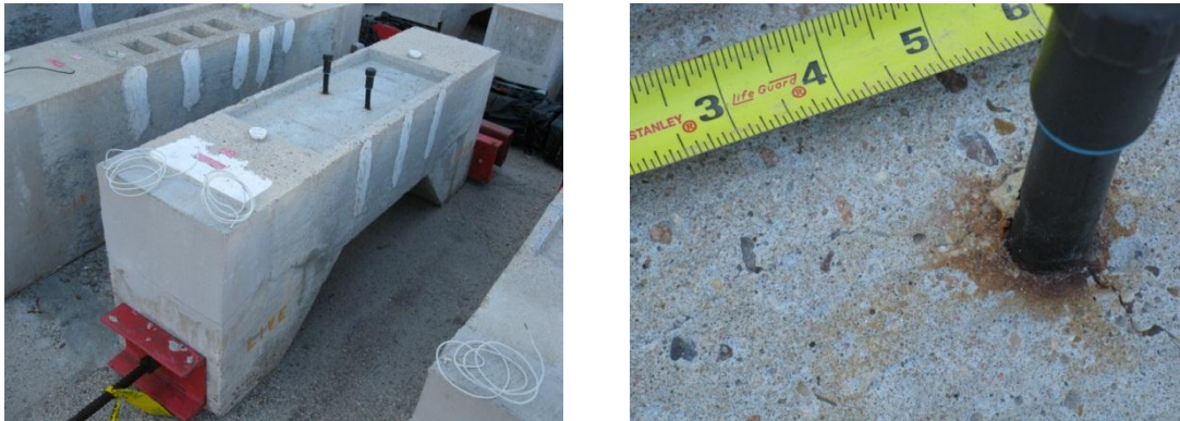
Figure 5.43: Specimen 2.2 Overall (Left) and Corrosion Stains Near Grout Vent (Right)
