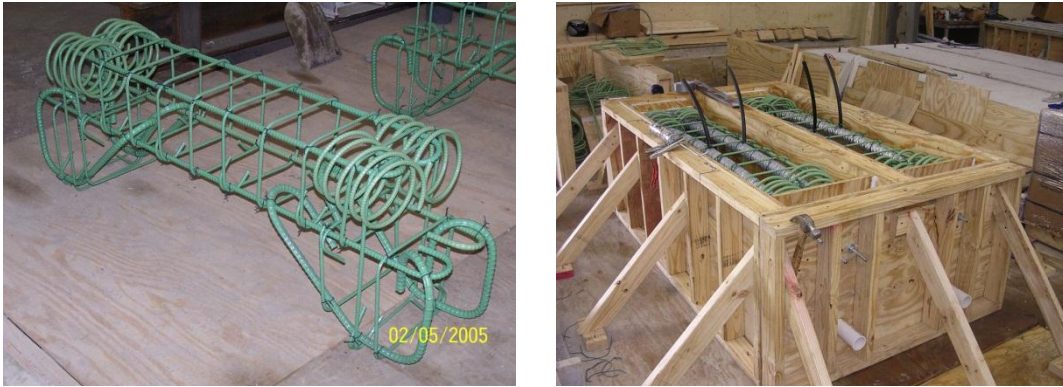
Figure 2.5: Epoxy-Coated Rebar Cage (Left) and Completed Reinforcement Cage with Ducts in Formwork (Right) 7
