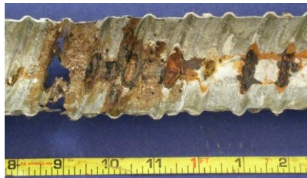
Figure 5.35: Specimen 1.2, Area Loss and Large Void on Top Inner Surface of North Duct
