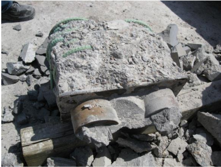
Figure 5.5: Partially Chipped Anchorage Block
