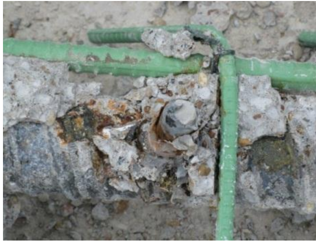
Figure 5.44: Specimen 2.2, Corrosion Staining Under North Grout Vent
