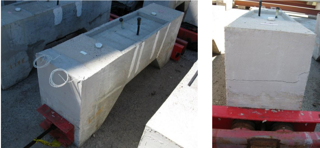
Figure 5.52: Specimen 2.4 Overall (Left) and Cracking at Dead End Pourback (Right)
