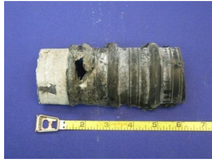
Top of South Duct
