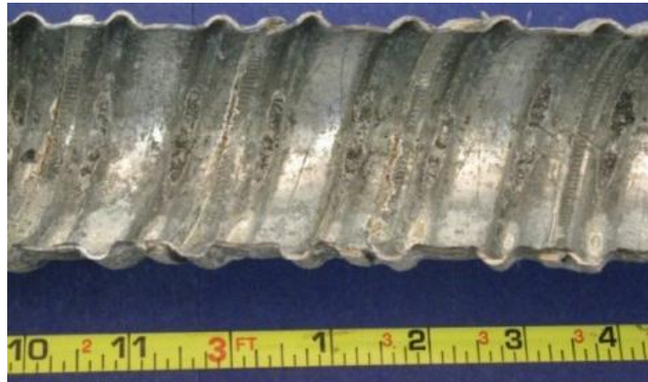
Figure 5.46: Specimen 2.2, Discoloration Inside South Duct Showing Signs of Cracked Grout
