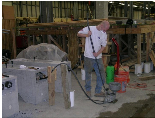
Figure 2.7: Grouting in Progress 7
