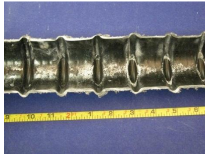
Top of South Duct
